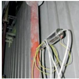
Adsorber / flue gas cleaning
